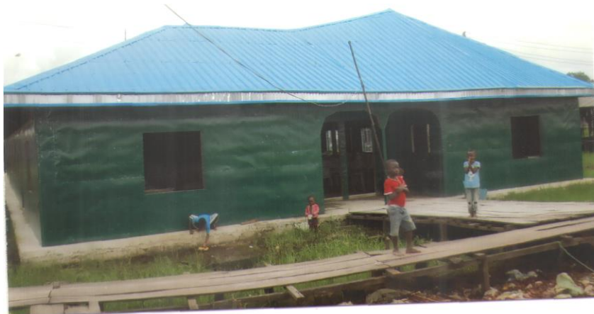
Figure 5: Current Auditorium of the First Baptist Church, Opuama
